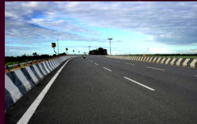
4.5 KM Alternate Link Road planned to ease congestion on Mathura Road & Kalindi Kunj.
