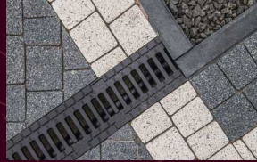
Drainage & Waterlogging Infrastructure Upgrades for improved monsoon resilience.
